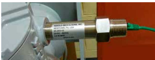
INSTALLED BECK MODBUS TCP ADAPTER
