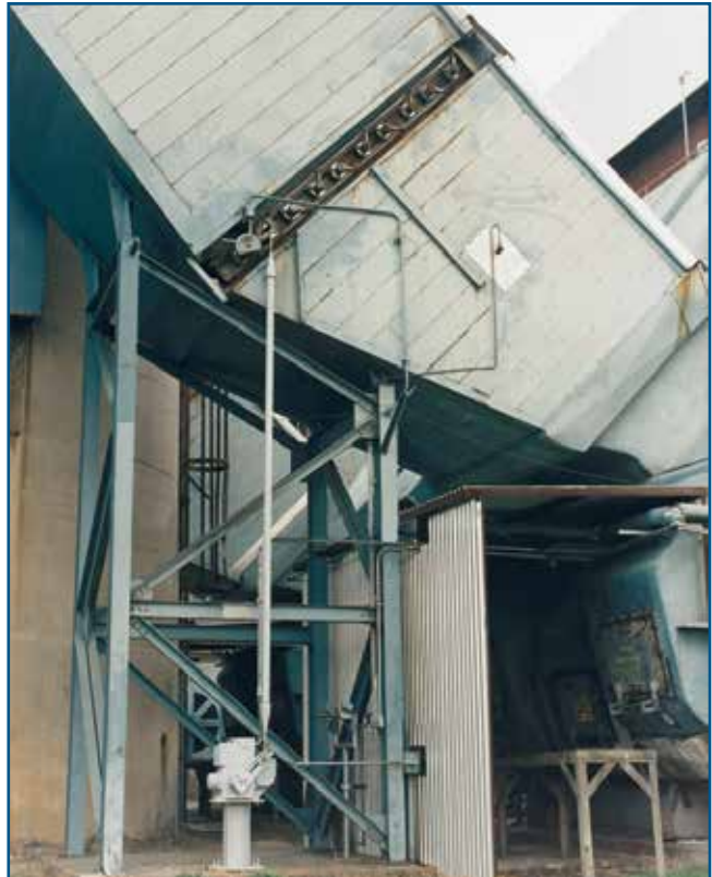
Beck actuator on a louver damper.
