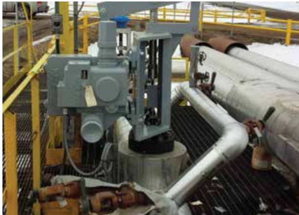
Figure 3. Actuator and fulcrum lever mounting assembly.
